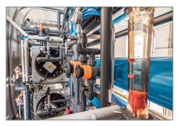
The technology can be installed in a space-saving and effective way even in the smallest area. All plant components for complete water processing can be accommodated in one container. This transportability allows decentralized use in e.g. work camps.
